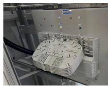
Splicing side of module
